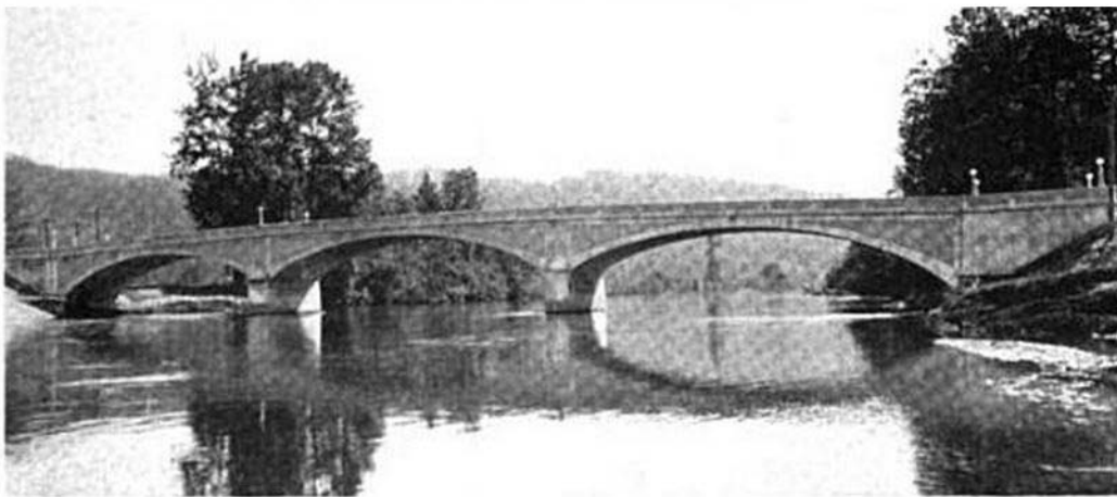
The stately strength of the Sunset Highway bridge as it crosses the Snoqualmie River at Falls City, is strikingly illustrated in this photograph.
