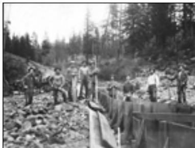
*Cover - Miners And Flume. The picture, taken about 1900 near Liberty, shows how gold was recovered from stream beds when there was only hand tools to get the job done. Dirt, gravel and gold was shoveled into the flume where water then washed the dirt and gravel away leaving the heavier gold behind in the riffles in the bottom of the flume. None of the miners in the picture have been identified.*
